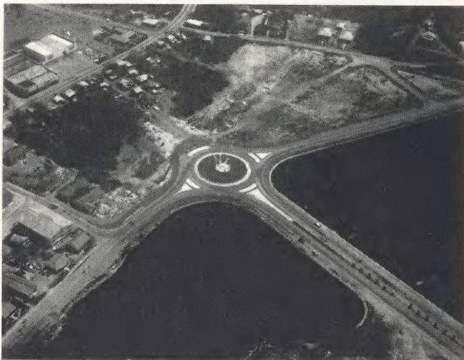
An example of modern road-building.
